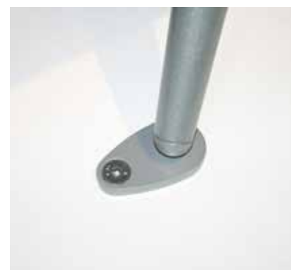
Floor fixings detail
